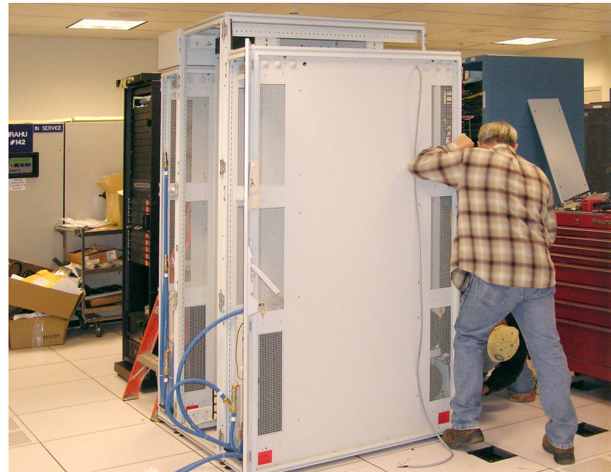
Joining the LCP to Equipment Enclosure
