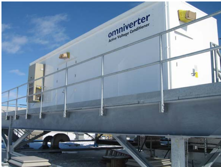
Apotex Inc 4800kVA AVC installed on the roof.
