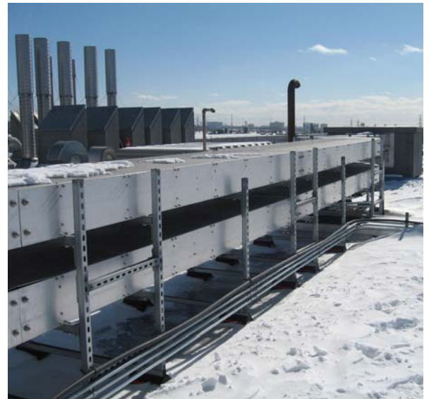
Apotex Inc 4800kVA AVC installed on the roof.
